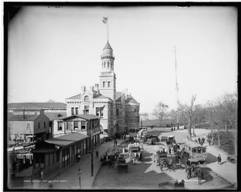
Barge Office, Lower Manhattan c. 1890 5
